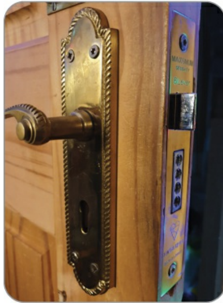
Figure 2-8: A mortise lockset installed in a door
